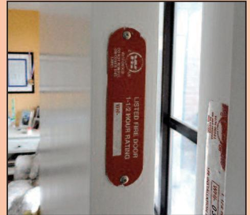
A fire door is a door with a fire-resistance rating (sometimes referred to as a fire protection rating for closures) used as part of a passive fire protection system to reduce the spread of fire or smoke between compartments and to enable safe egress from a building or structure or ship.
