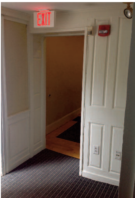
Door widened to accommodate wheelchair access
