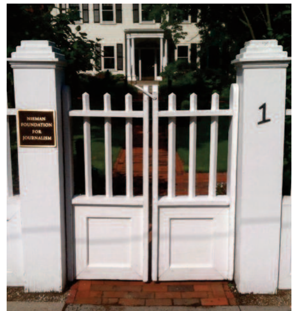
Gate is reconditioned to wing like it was as good as new.
