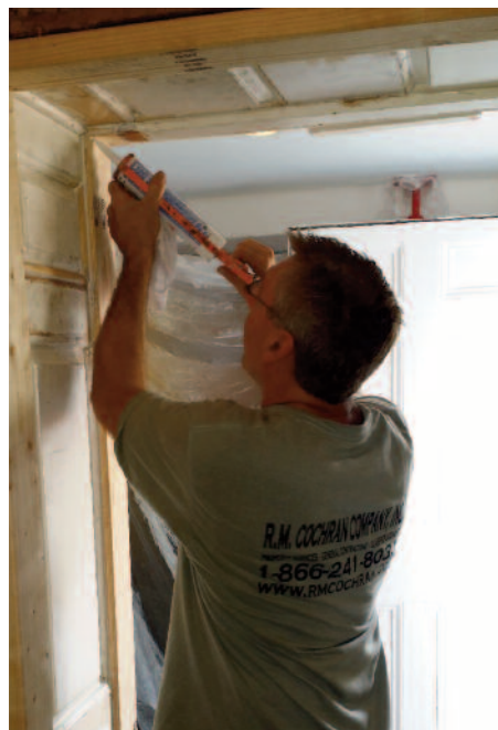
One of our carpenters working on expanding doorway
