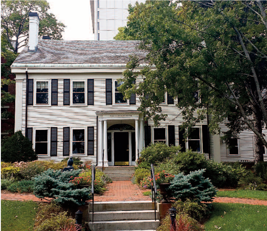
We installed brand new storm windows to help keep the heat in!
