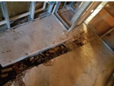
Another component of the Broadway Project is the conversion of unit IA from a standard unit to an ADA unit. This conversion required significant coring to move re-organize the kitchen and bathrooms.
