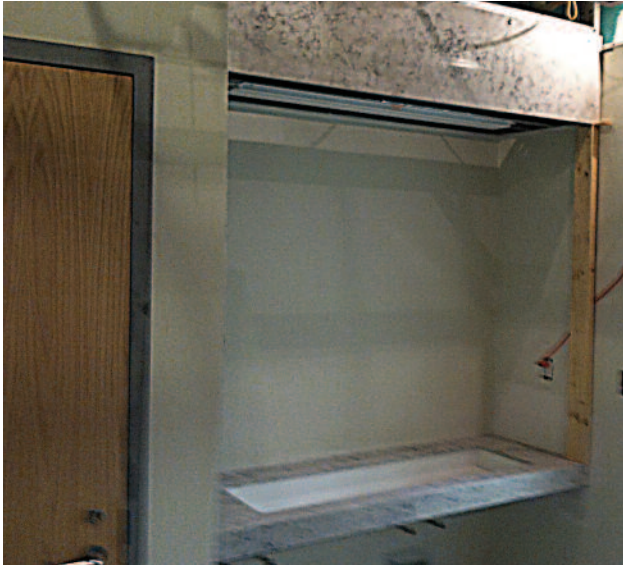
The installation of the custom corian sink and counters.
