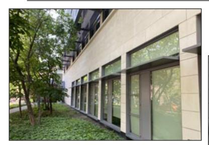
RM Cochran finished up the exterior cleaning and maintenance project on this Harvard property. The entire building was pressure washed, rusty areas treated and primed and most external metal
