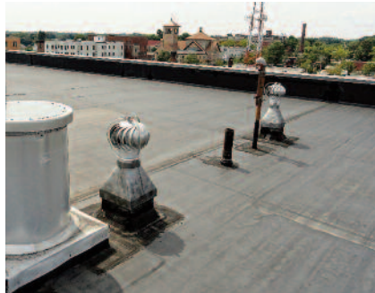
Another area of focus is where roof penetrations have occurred. Vents and AC units installed after the original roof can be problematic
