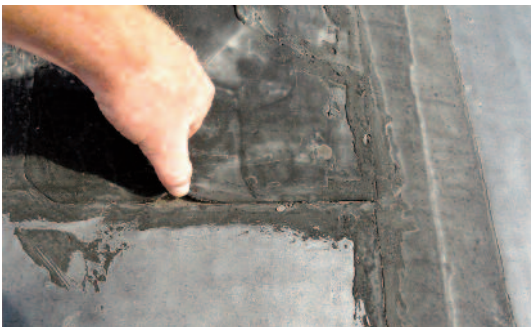
Inspections usually start at the seams where water penetrations can occur
