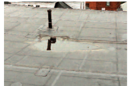
Ponding, a problem on flat roofs, is likely to lead to leaks and is typically symptomatic of additional roofing problems.
